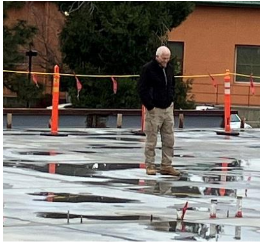
January 19, 2024: Greg Kidder inspects the newly poured slab:
